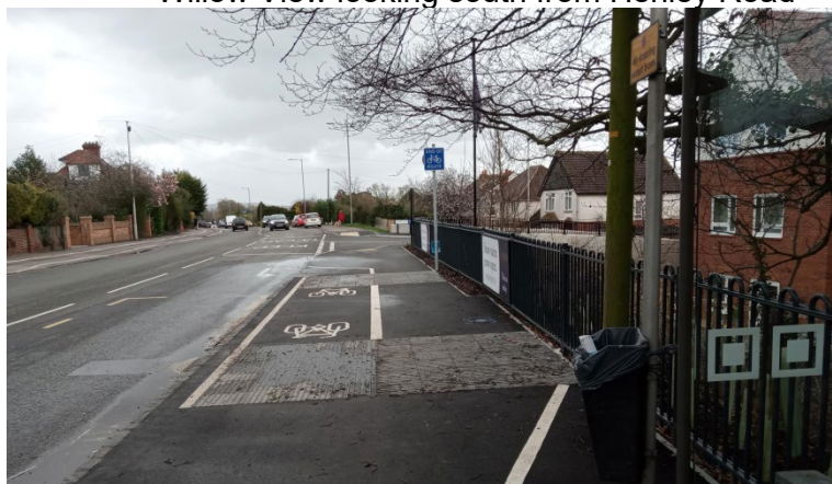
Officer photograph 23/03/2023 – recently installed pedestrian/cycleway to west
